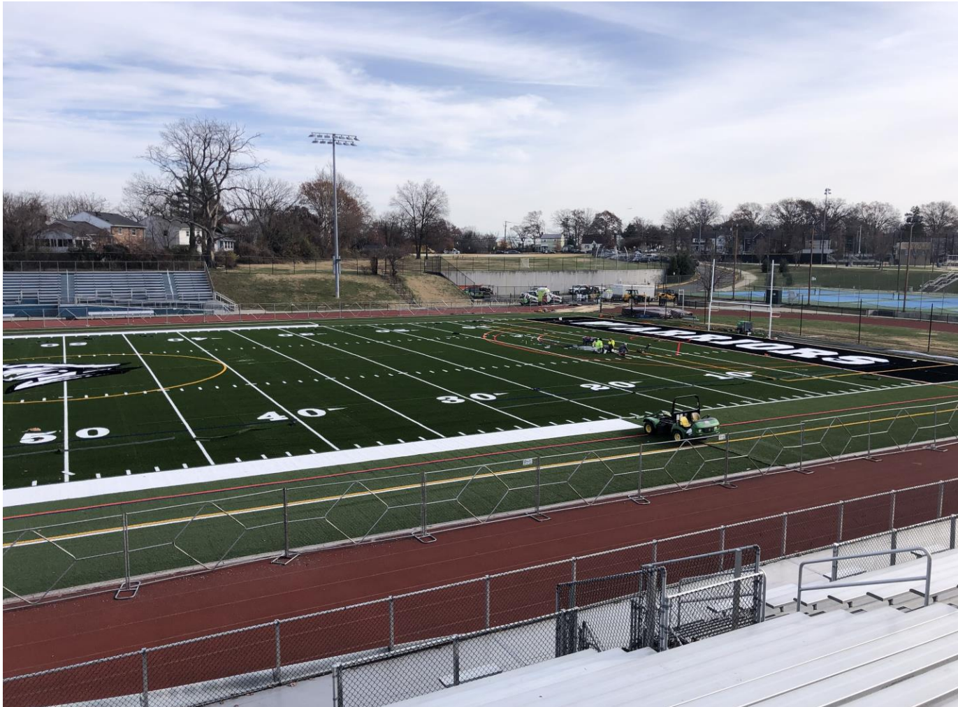
Wakefield HS Synthetic Turf Replacement Project Early Winter 2022
