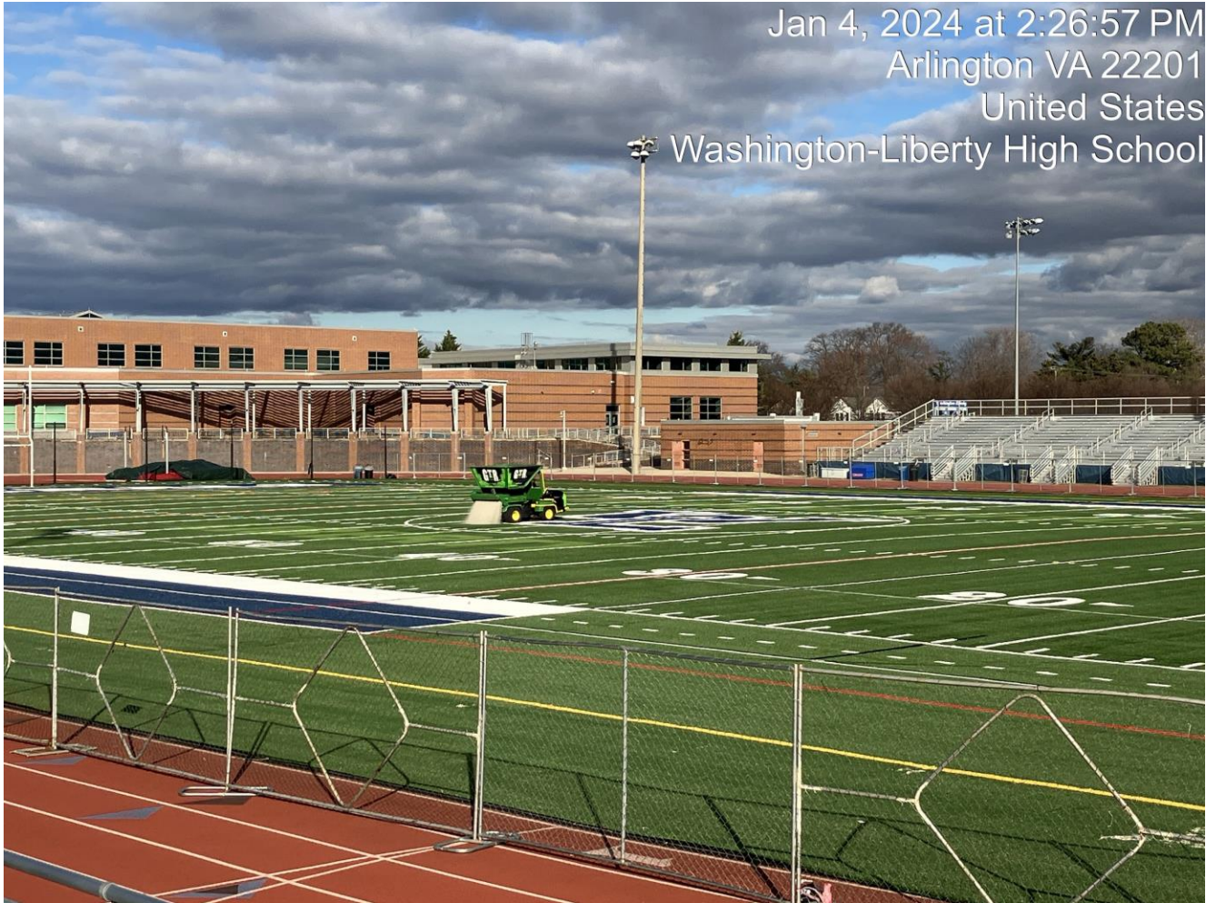
Washington-Liberty Synthetic Turf Replacement Project Early Winter 2024
