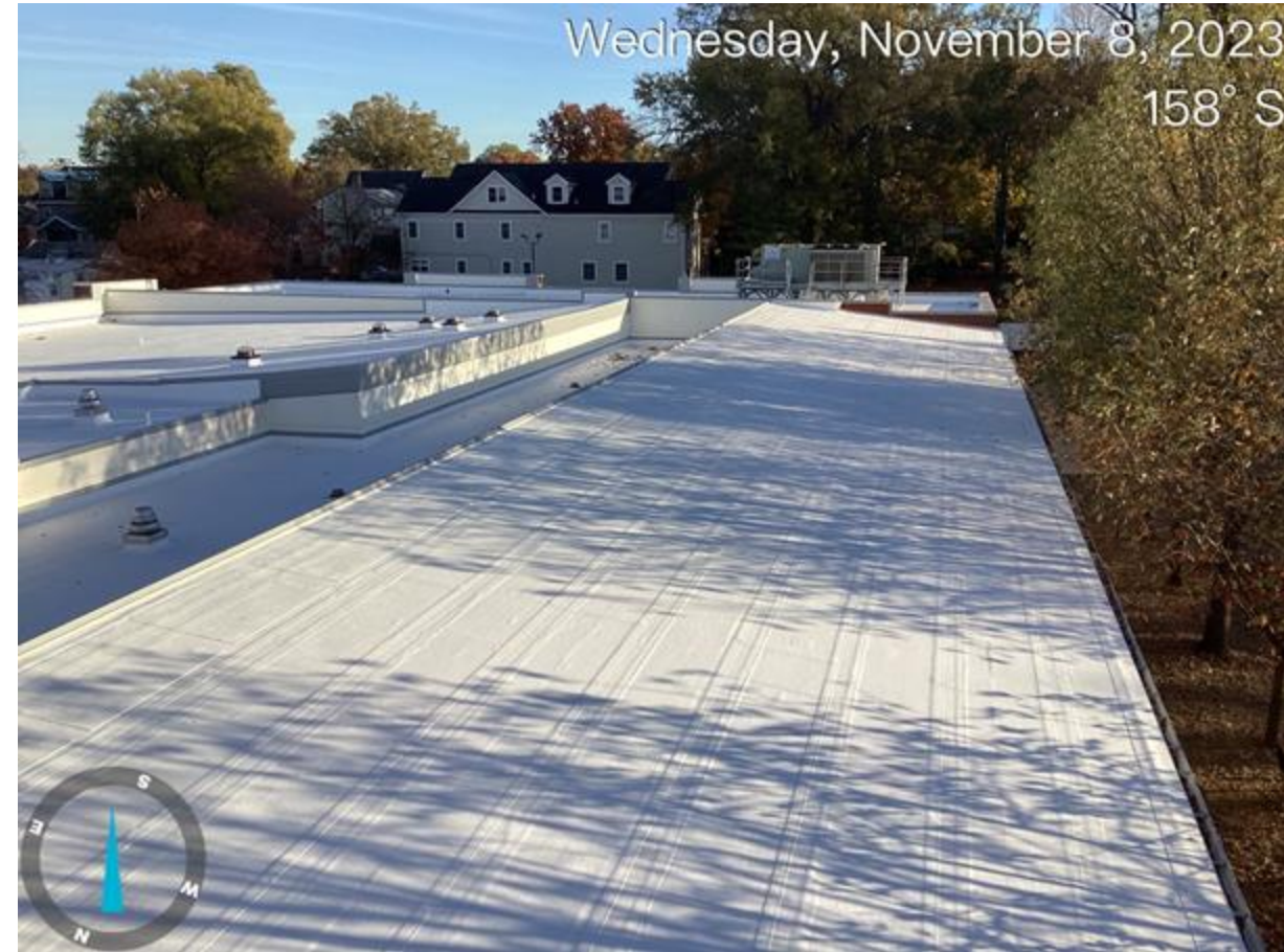
Randolph Roof Replacement Project Fall 2023
